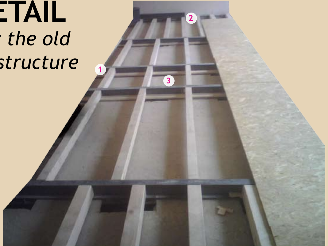
1 FIX OF THE IPE 120 BEAM PERPENDICULAR TO THE MAIN WALLS
