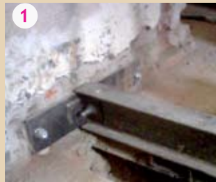
1 FIX OF THE IPE 120 BEAM PERPENDICULAR TO THE MAIN WALLS
