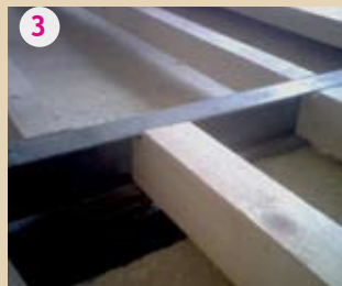
3 FITTING WITH WOODEN JOISTS AND THE IPE
